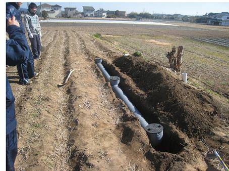
**Fig. 6** The experimental pipe before buried in the ground.
